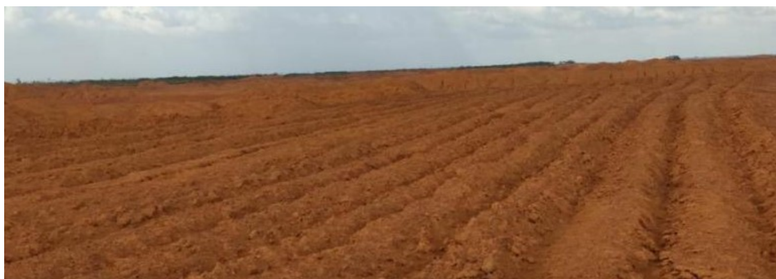
Figure 6. Soil decompression activity with a scarifier, after topographic recomposition with residual soil.
